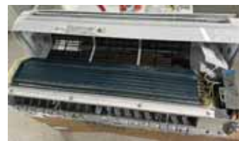
3. Remove the cover by removing these 10 screws.
