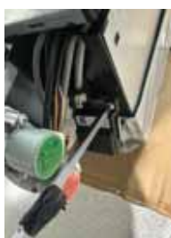
5. Remove leak sensor.
