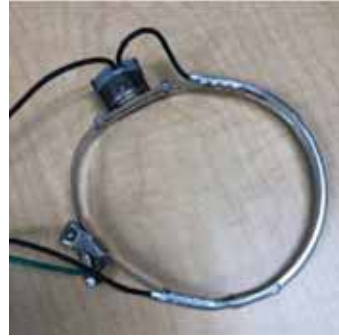
Figure 37. Checking Crankcase Heater Thermostat
