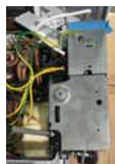
4. Remove the electrical box cover.
