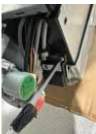
5. Remove leak sensor.
