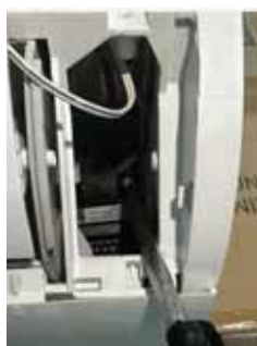
3. Remove leak sensor.
