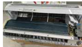
3. Remove the cover by removing these 10 screws.
