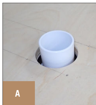
FIG. 5. Cut the coupling (A) and the PVC tubing (B) flush with the countertop.
