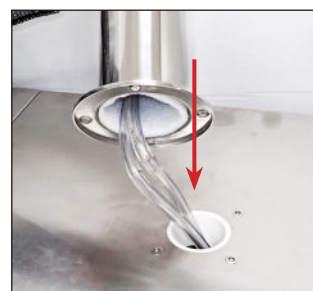
FIG. 2. Thread the draft standard lines into the appliance.
