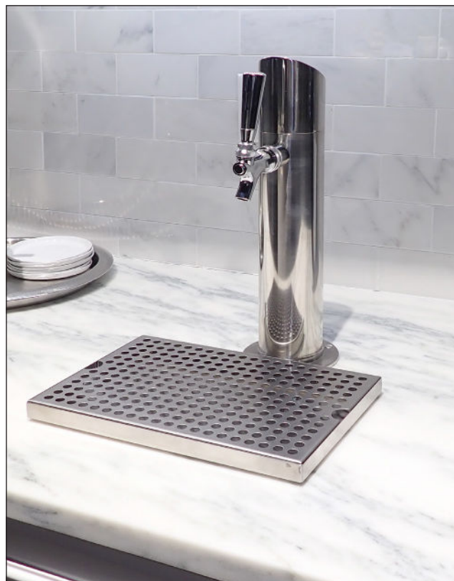
FIG. 1. Example of countertop draft standard installation.
