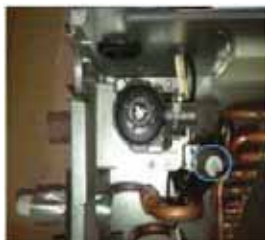
Built-In Condensate Pump and Float Switch
